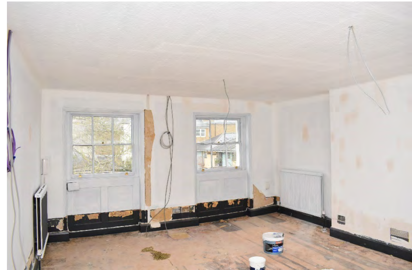
Plate 53: No 16 Second floor rear room
