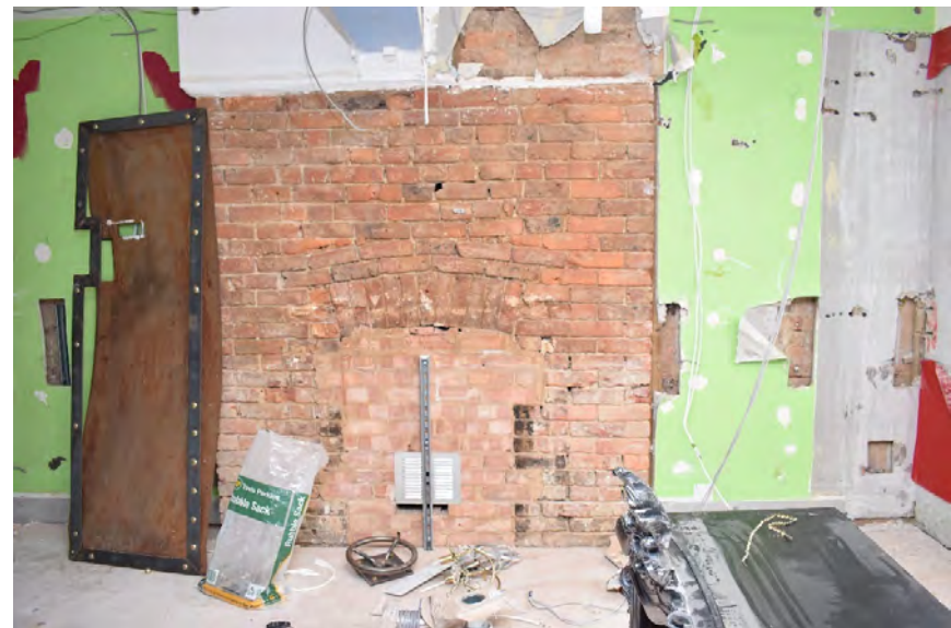
Plate 18: No. 16 First floor bricked up fireplace.
