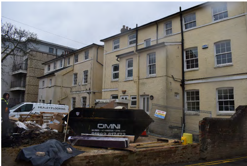
Plate 52: Rear of Nos 16-22
