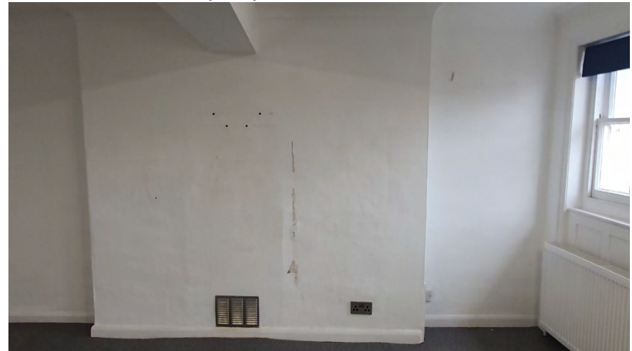
Plate 41: No. 18 Second floor front room
