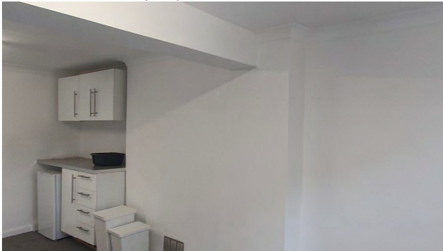
Plate 43: No. 18 Second floor rear room
