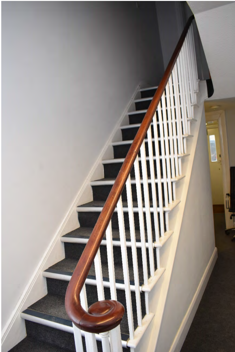
Plate 16: No. 16 Ground floor stairs
