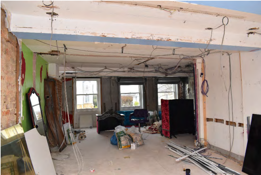
Plate 19: No. 16 First floor room
