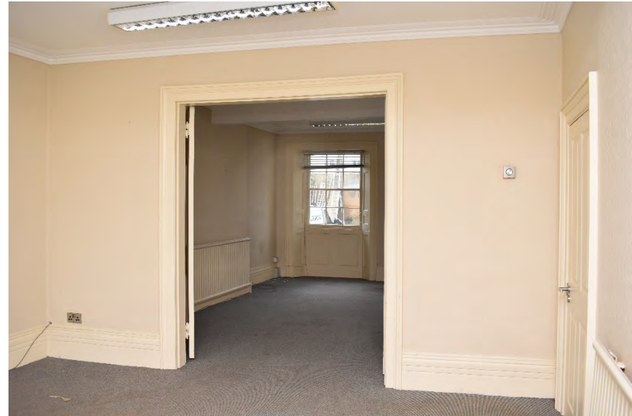
Plate 30: No. 18 Ground floor dividing wall
