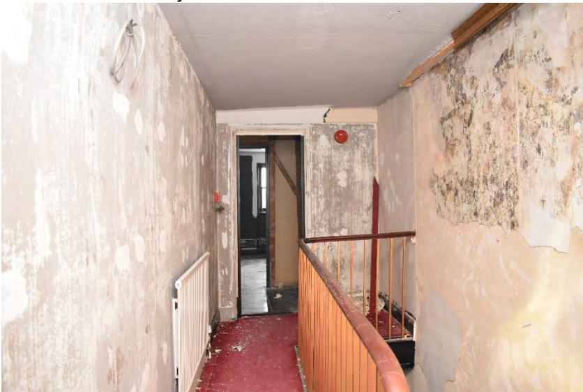
Plate 20: No. 16 Second floor landing
