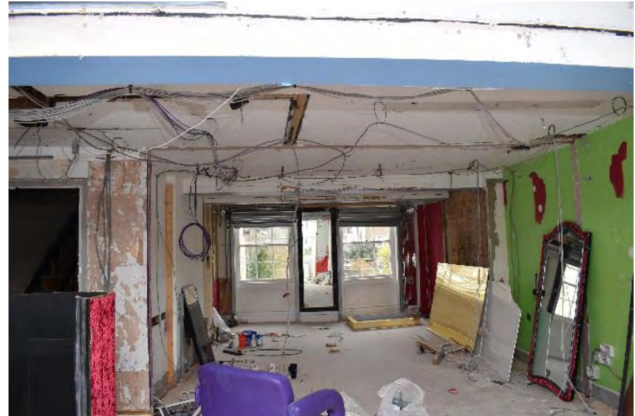
Plate 17: No.16 First Floor
