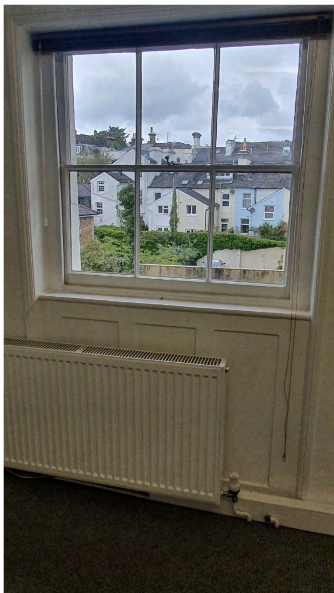
Plate 45: No. 18 Second Floor rear room
