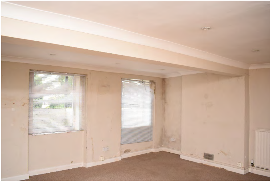
Plate 47: No. 18 Basement room (facing)
