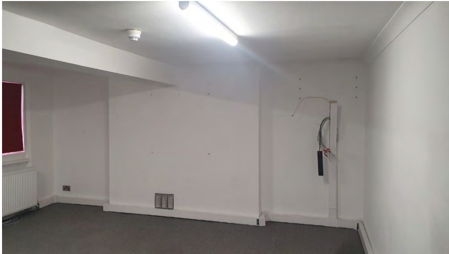
Plate 42: No. 18 Second floor front room
