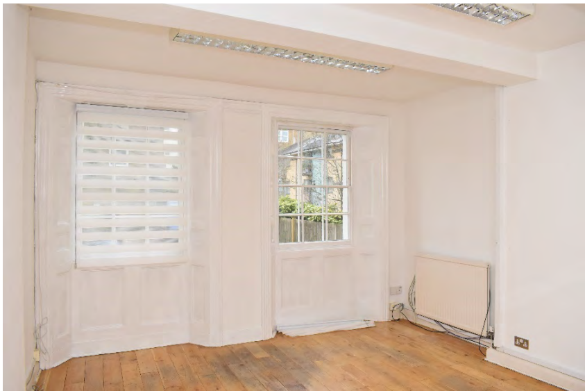
Plate 14: No. 16 Ground Floor rear room
