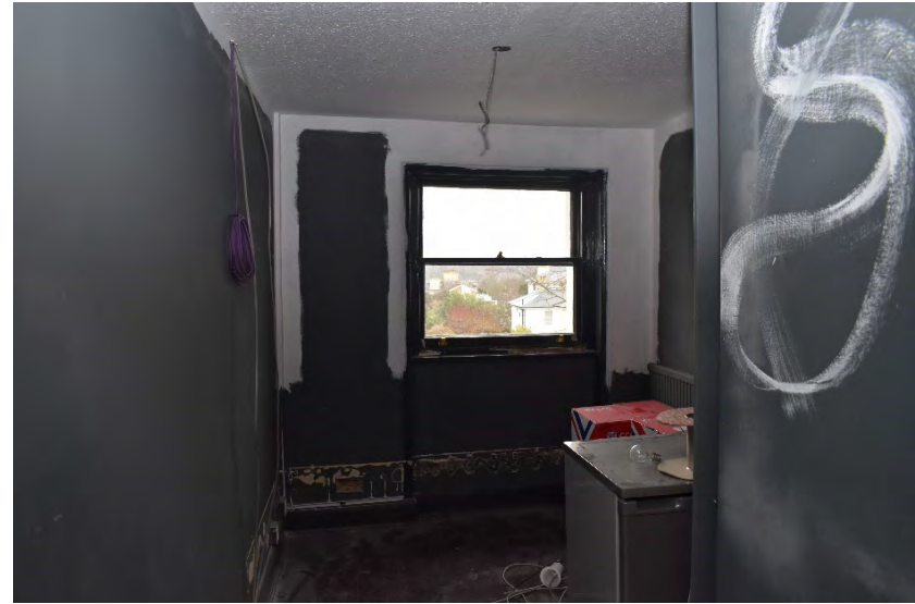
Plate 21: No.16 Second Floor front western room
